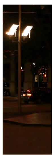
Currently, the only permanent lighting in the 12,000 sq. ft. central plaza is around its perimeter, where 8 poles are mounted with 2 lights each. The lights are directed UP onto diffusers that are supposed to reflect the light onto the area below. In actuality, this system fails to provide ample illumination.
